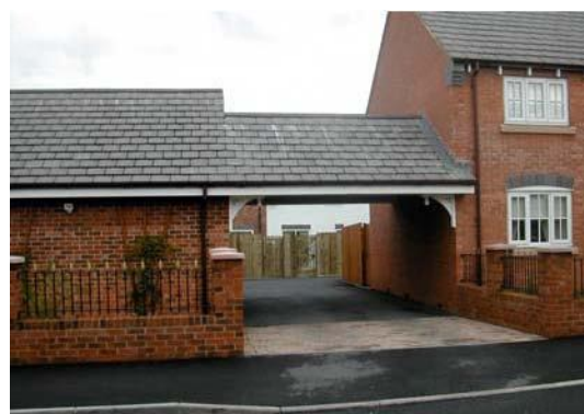
Rear courtyard parking
